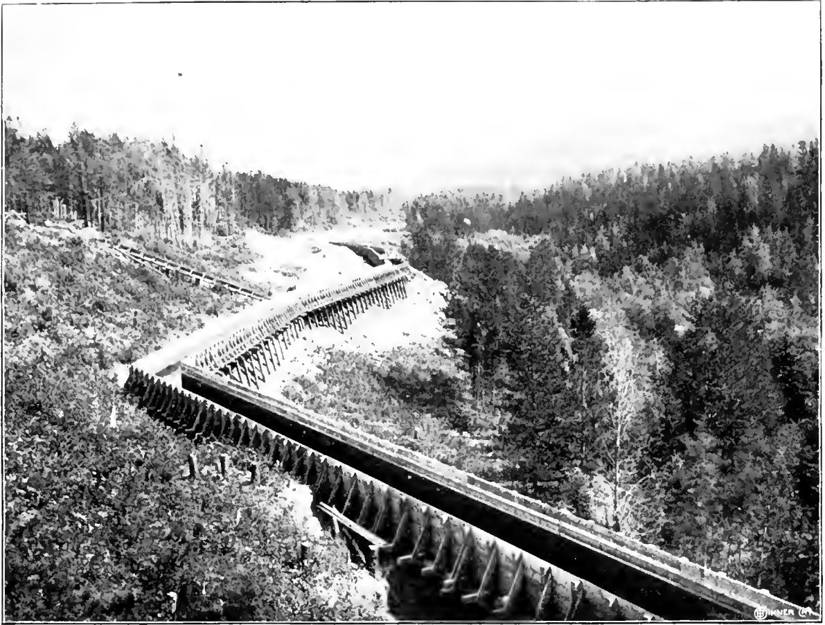
CONSOLIDATED CARIBOO HYDRAULIC MINING CO.'S FLUME.
